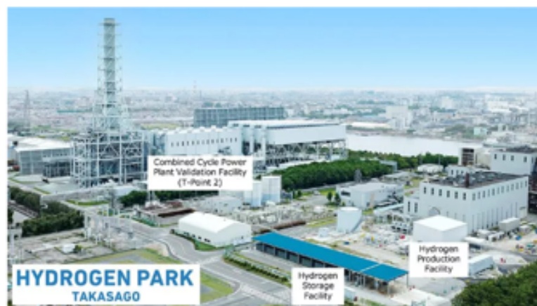
Hydrogen Production/Storage Facilities and T-Point 2 in Takasago Hydrogen Park
